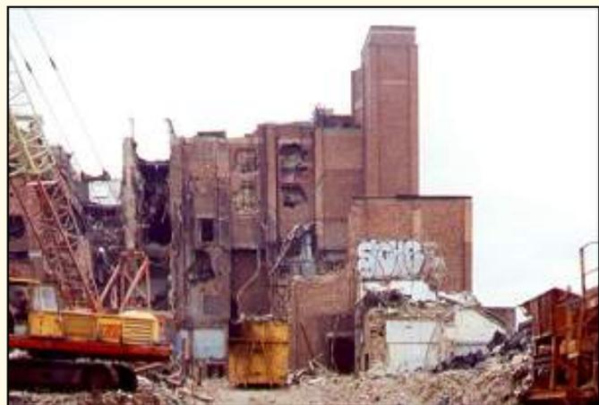
North Block rear section (adjacent to railway). Large holes have been knocked in the brickwork of Studio D by the demolition ball, revealing the interior wall insulation.
