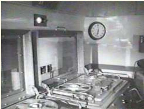
The BTR2 recorders, which superseded the BTR1, both made in England by EMI, became an "industry standard" in the BBC.
