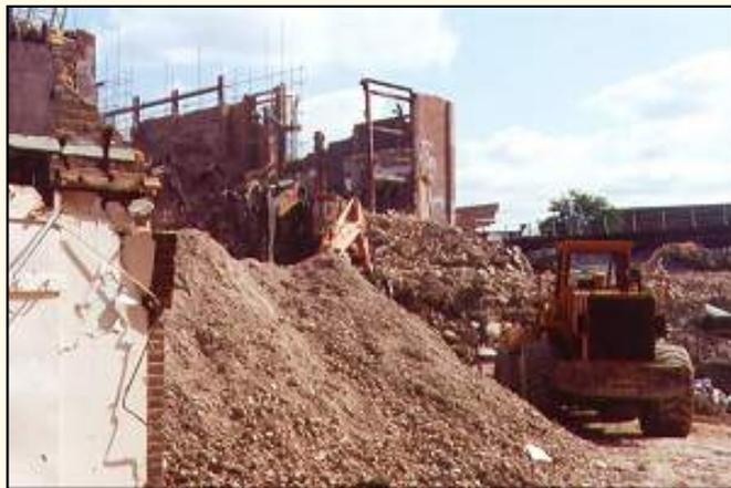
The rear wall of North Block was too close to the railway line to be knocked down, so it had to be taken down by hand.
