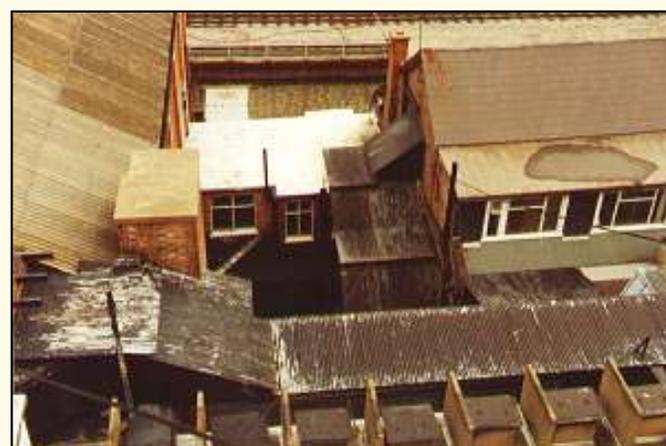
Film Vaults (7th floor). Note the flame trap walls between each vent hatch.
