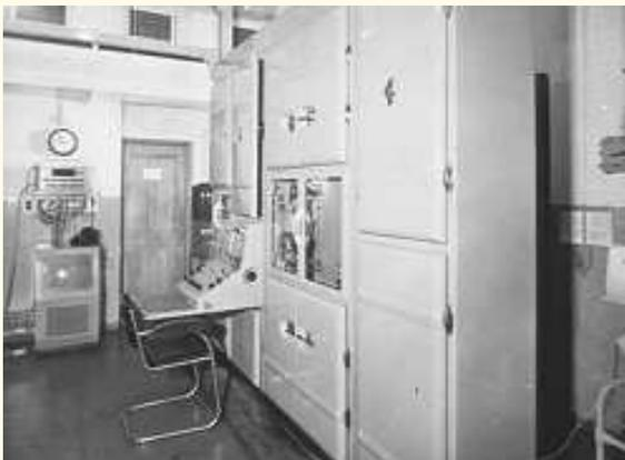
There were two EMI telecine machines at Lime Grove, they weren't as good as Cintel (although to say so could provoke heated arguments.....), and they looked as if they'd been built using kitchen cupboard and refrigerator doors..... and on these we ran the morning Demfilm for a period until a single Cintel machine was temporarily hired, just to run the Demfilm, thus freeing the EMI machines for other purposes, studio rehearsals for example.
