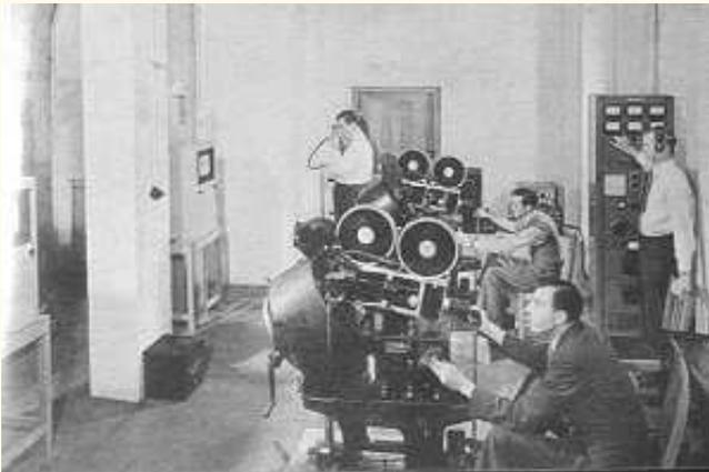
Even before the Suppressed Frame Telerecording system, first used for the Coronation, in 1953, there was a tv recording system at AP. It was housed in a basement room, just along a corridor from Central Telecine, and comprised a pair of Mechau machines looking at good quality monitors.
