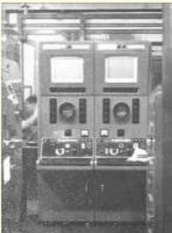
Although well built and giving superb pictures, they were designed by engineers and not operational staff, so sitting at the control position, the picture monitors were right up at the top, and so the operator tended to get a stiff neck from looking up at them.....
