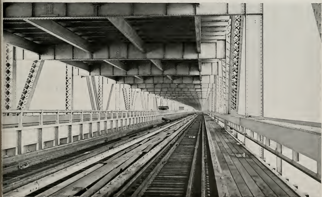
This view looking down the East Bay Crossing shows ties and tracks in place.
