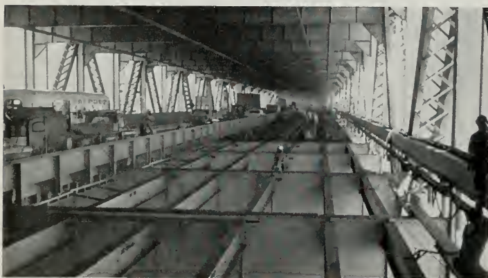
A section of the lower deck of the Bay Bridge during reconstruction with the railway tracks removed.
