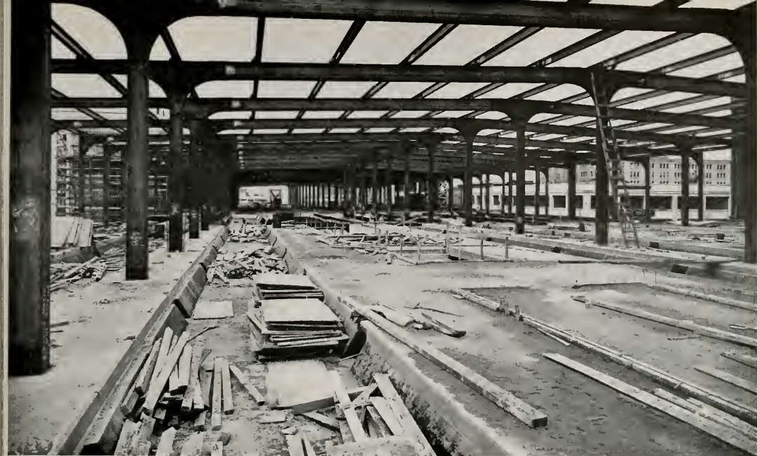
Trains will roll in the San Francisco Terminal over six tracks arranged in pairs. This view of the elevated track level also shows the roof steel just erected.
