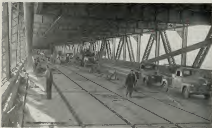
Deck slabs in place ready for pouring of concrete into the joints.
