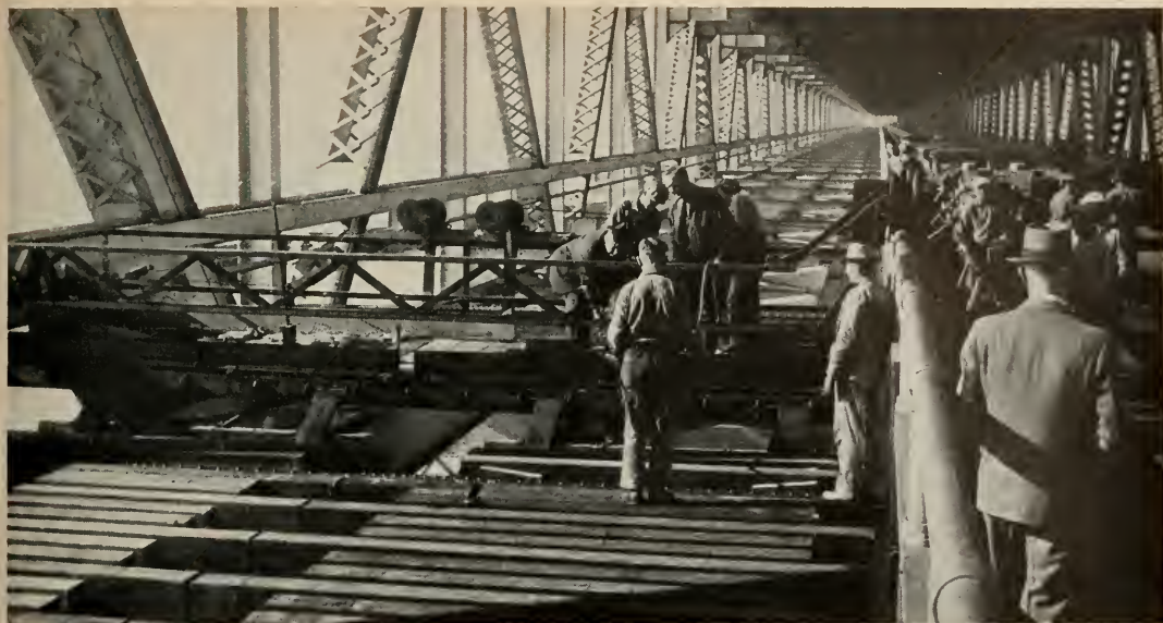
This picture shows the laying of ties for the San Francisco-Oakland Bay Bridge railway system at easterly edge of span.
