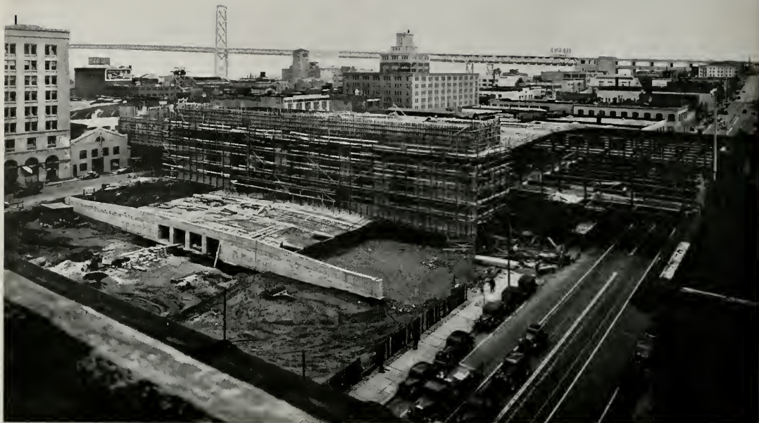
The San Francisco Terminal, facing Mission Street, showing the center unit well under construction. Street car ramp in the foreground. East and west units not visible.
