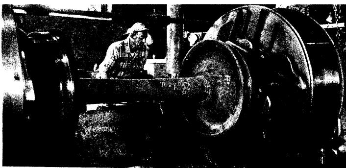
Machinist Victor Dyson grinds down a pair of wheels using the huge lathe in the system wheel shop. The facility works on all passenger, freight and locomotive wheels.
