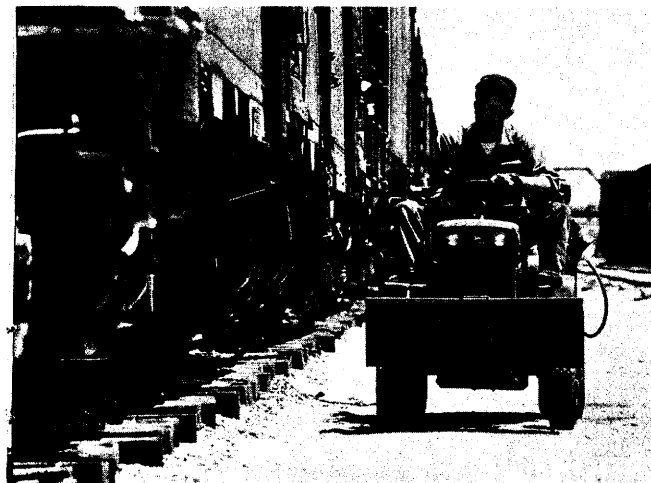
Machinist Victor Dyson grinds down a pair of wheels using the huge lathe in the system wheel shop. The facility works on all passenger, freight and locomotive wheels.
