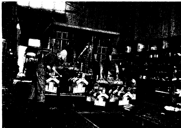
Herington/ G. F. Duncan, motor car mechanic, works on a Jackson tamper. Herington is the maintenance of way equipment and motor car repair center for the system.
