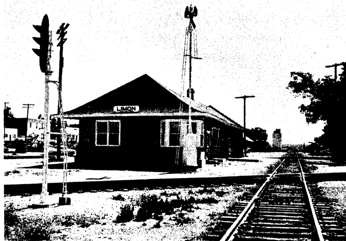
Limon/ Rock Island trains run over the Union Pacific from Limon to Denver. Westbound Rock Island trains swing behind the station and join the UP mainline at the left of the picture.
