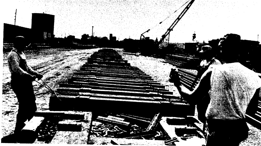
Des Moines is one of two locations on the Rock Island where track panels are prefabricated in assembly line fashion. Ties are lined up on special forms, rails are placed on them and then spiked into place. The resultant panels are used for industrial sidings and emergency use.
